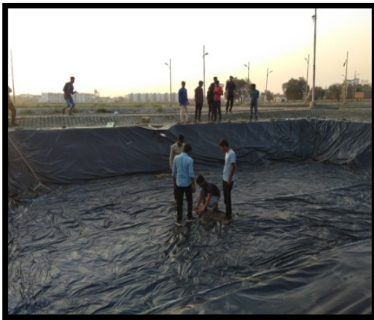
Laying of polysheet for fish culture
